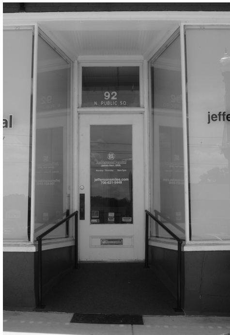
This door maintains its original form and design.
