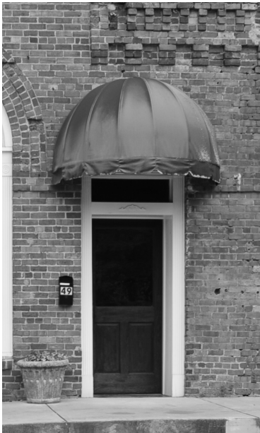
An example of an inappropriate bubble awning.
