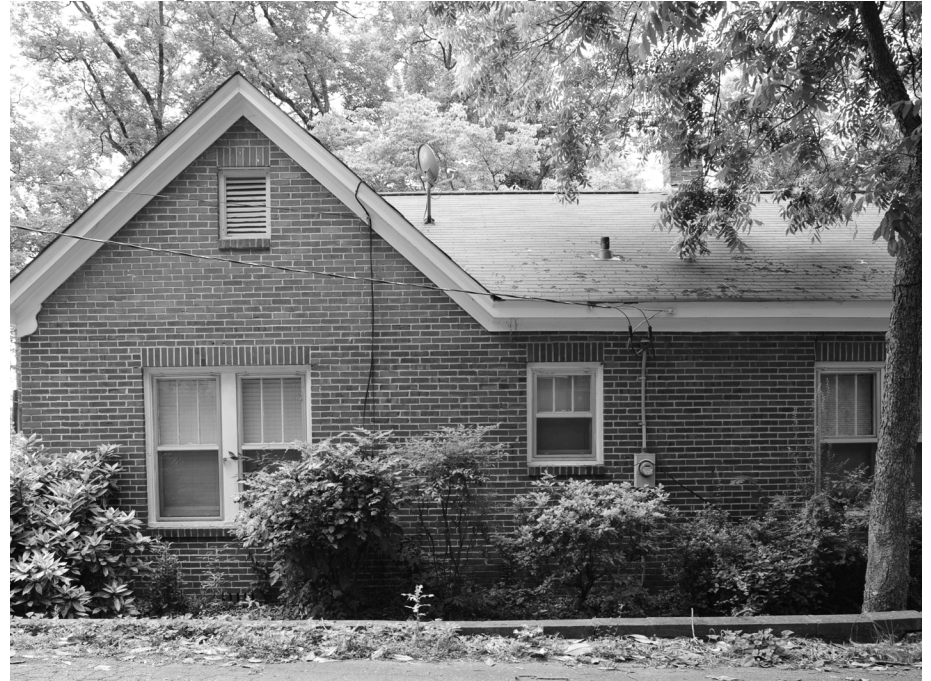
The satellite dish attached to this house is well hidden behind the roof line. This is the ideal placement as it cannot be seen from the front facade of the building.
