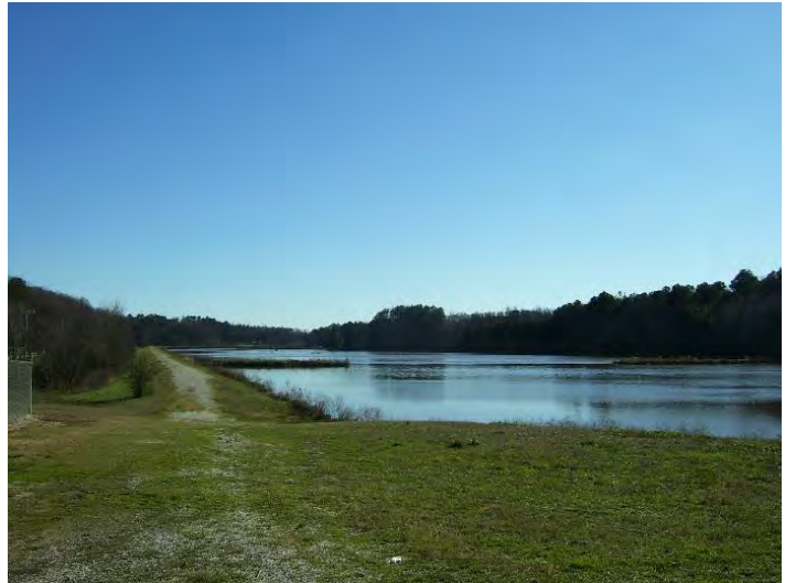
Curry Creek Reservoir
