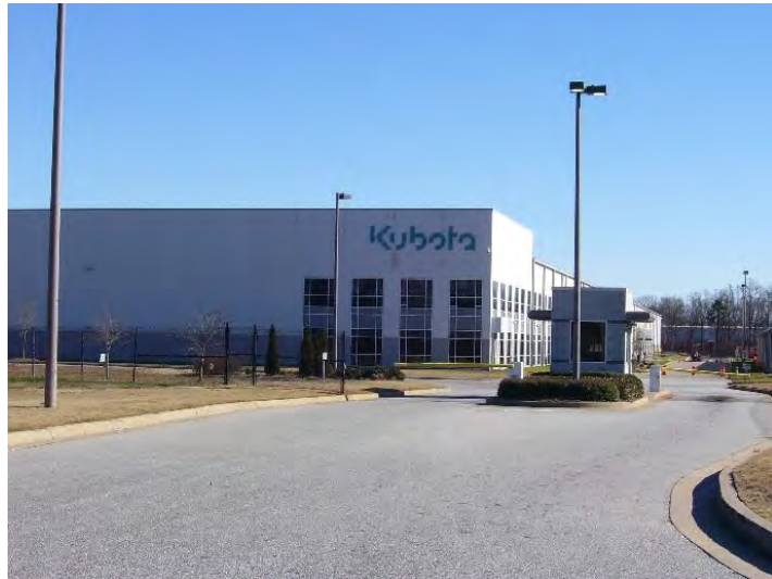
Kubota Building Addition
