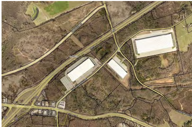
Warehouse construction has raised concern among the citizenry
