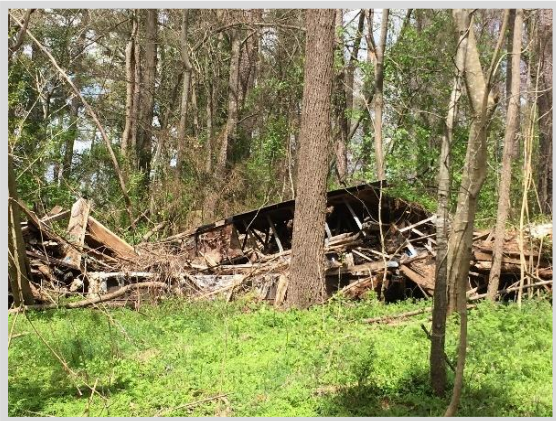
COLLAPSED STRUCTURE ON PEACH CIRCLE
