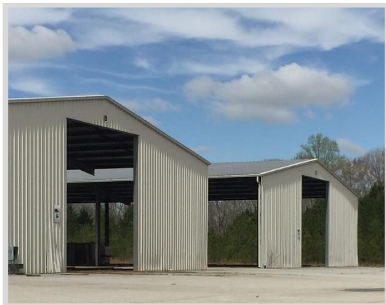
EMPTY WAREHOUSES IN THE CENTRAL JACKSON INDUSTRIAL PARK
